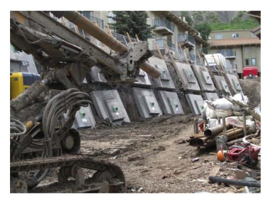
The enormous scale and depth of excavation is better seen in the next two photographs. The first was taken from what used to be the driveway in front of Building B. The second shows owner Eric Loeb and Hank Hays standing in front of (and dwarfed by) the shoring blocks, part of the MSE wall designed to hold the mountain behind us in place.
