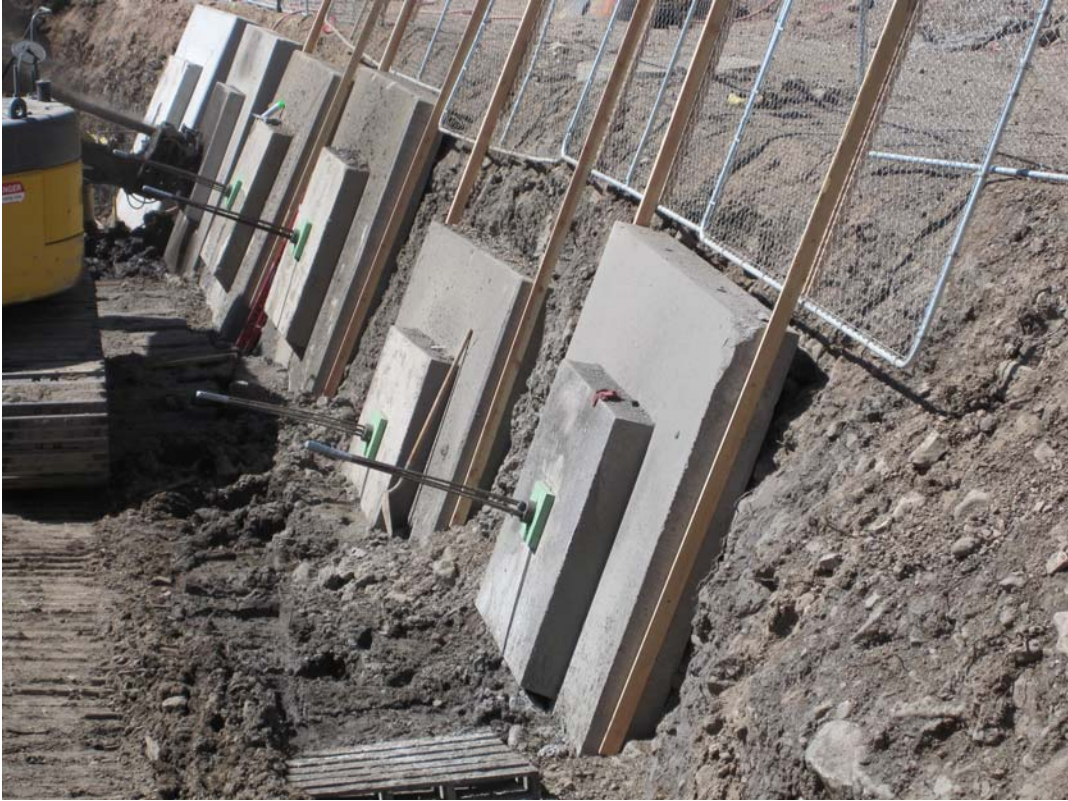
Above and below (closeup): Shoring blocks that have been anchored into place.
