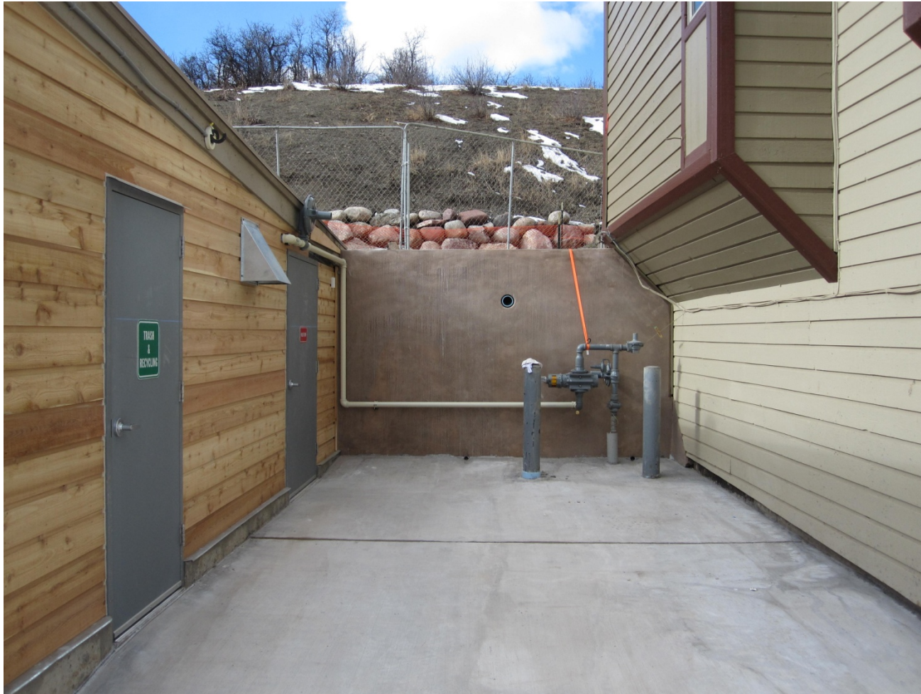
New Retaining Wall and dual-purpose shed housing boilers in back and trash/recycling dumpsters in front
