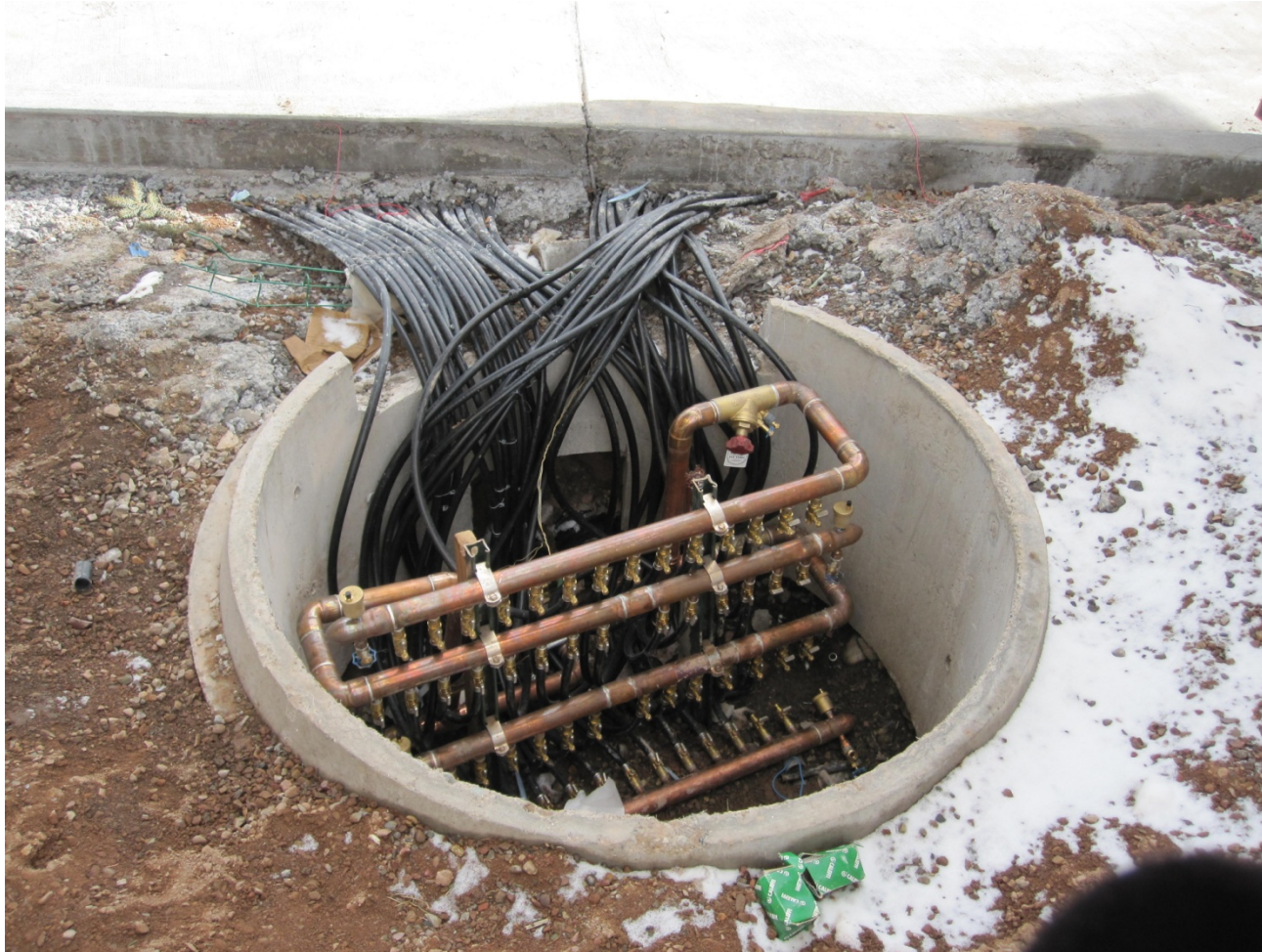
Controls for new Snowmelt System-6 miles of pipes under the driveway
